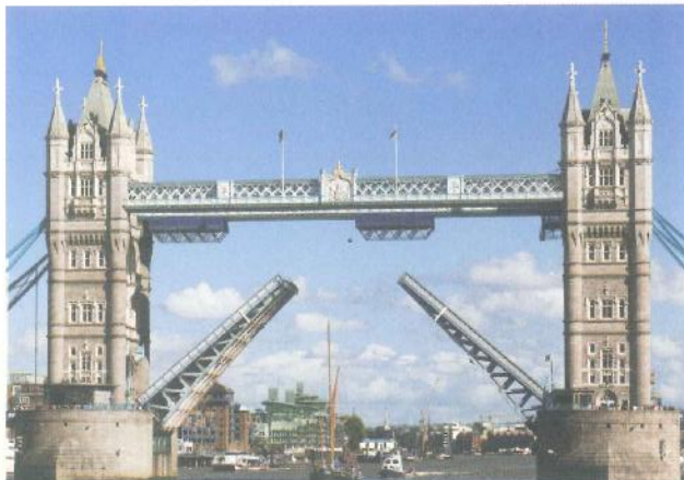
17 Tower Bridge – Londres (1892)
